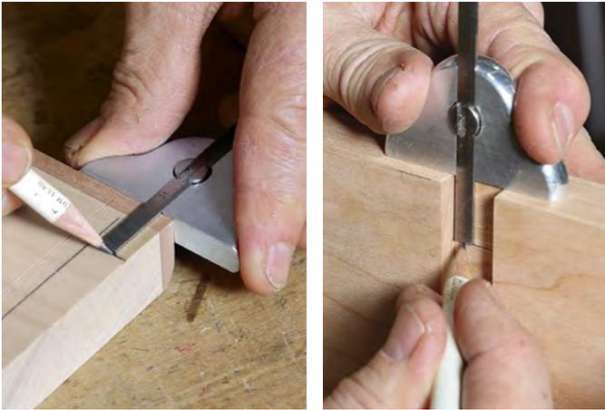
**Mark the dovetail and housing.** Use a depth gauge to mark the width of the dovetail both on the divider and the case side.
